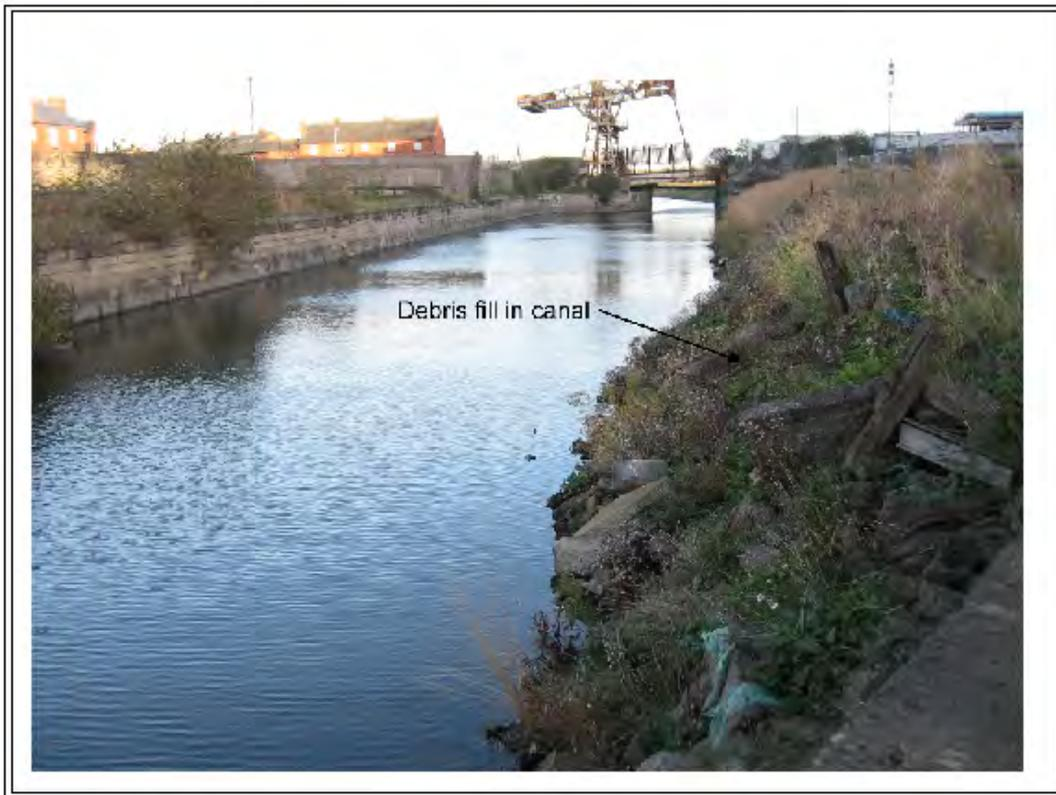
Plate 4: Example of material dumped in canal at Spencer Dock
